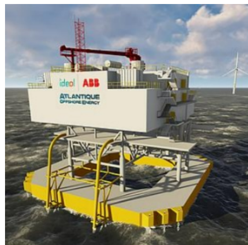
Figure 12 Floating offshore sub-station
